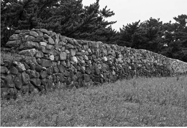
FIGURE 56. Partially reconstructed defensive wall in Fukuoka. Courtesy of Fukuoka Board of Education, photo by author.
